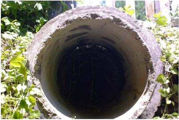
Separation of Outlet pipe behind 6613 Riverbirch Drive.
