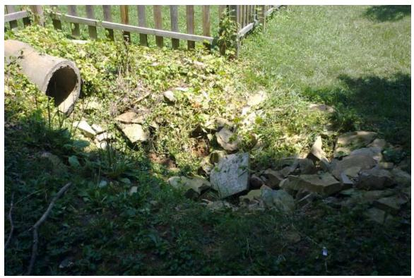
Outlet pipe and erosion problems behind 6613 Riverbirch Drive.
